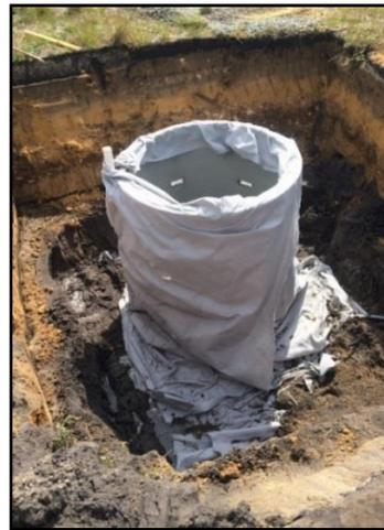
*Plates 1 & 2: Soakwell on concrete base lowered into excavated hole and wrapped in geotextile fabric, then backfilled to surface.*
