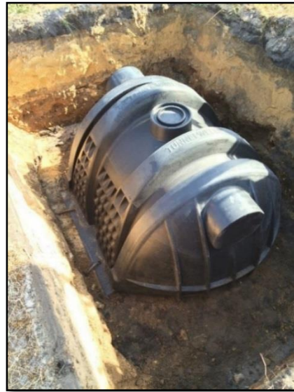
Plate 4: Tunnelwell in pit ready for backfilling.
